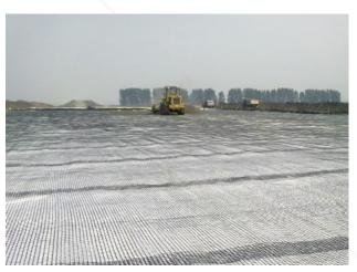
Geosynthetic materials are effective construction solution for waste landfills. The landfills for municipal solid waste (MSW) might be potentially dangerous not only for soils, but also for atmosphere and groundwaters.
